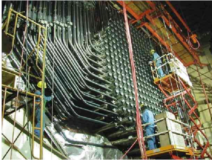
Figure 2 Feeder tube assembly on reactor face
