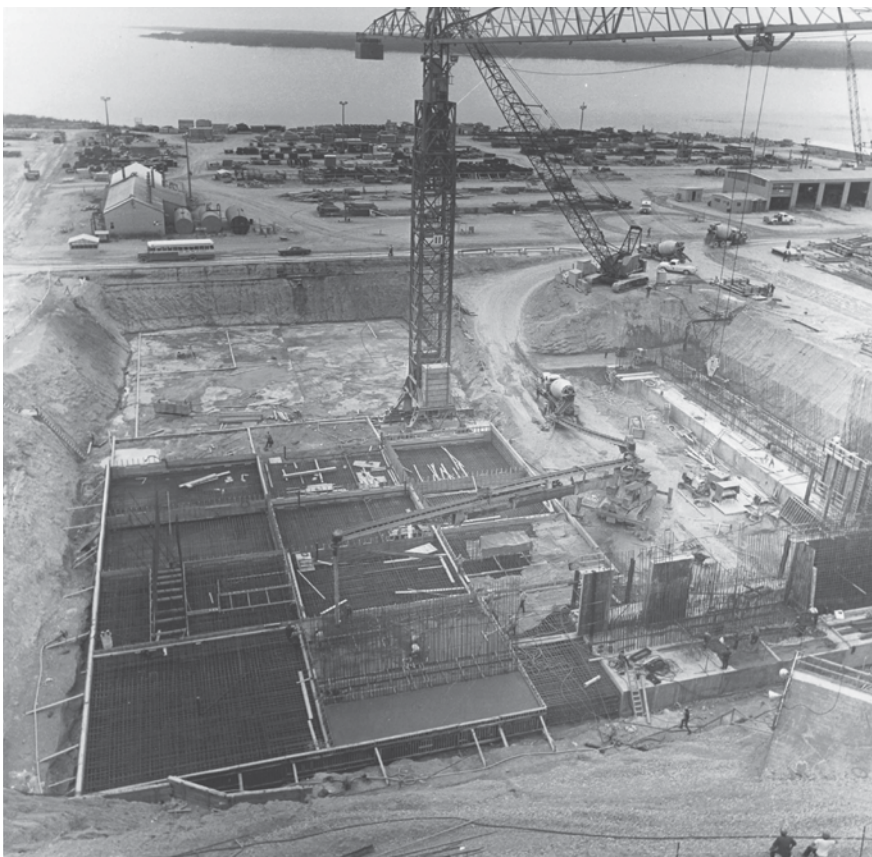
Preparing a reactor’s foundation
