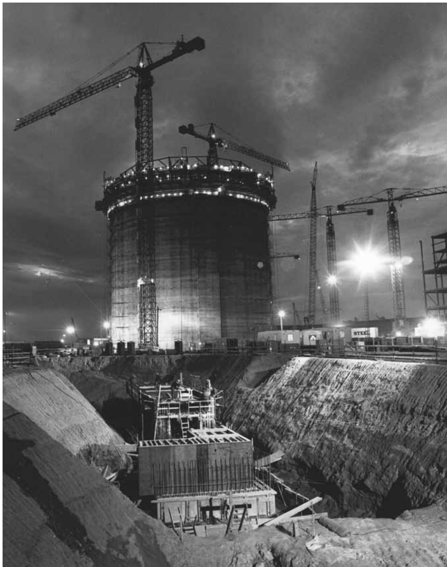
Wolsong construction by night
