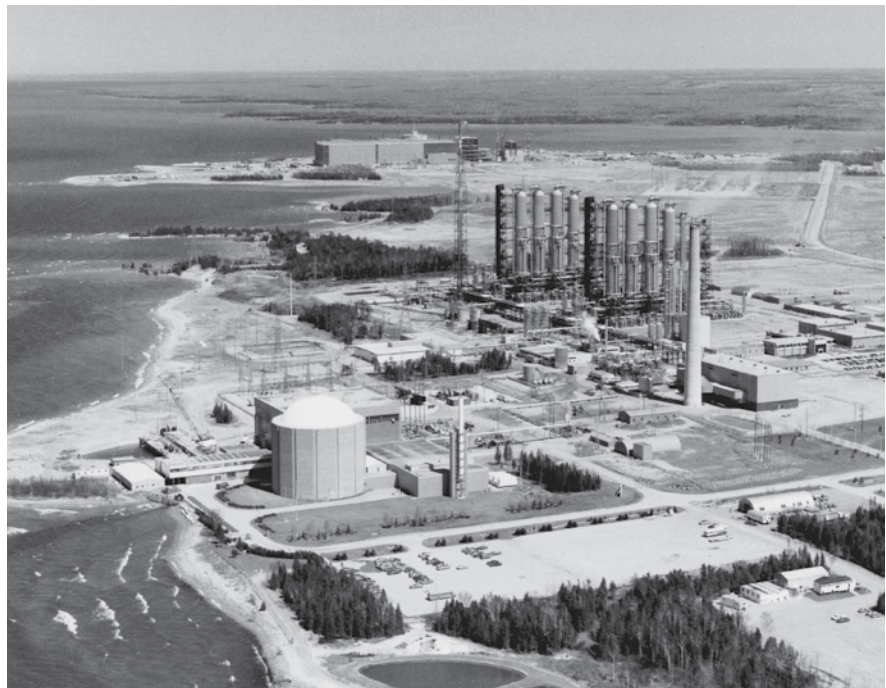
The Bruce heavy water plant, shown next to the Douglas Point reactor
