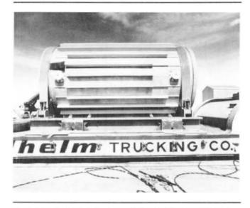
Figure 4: The third storage cask (MC-10) built by Westinghouse Electric Corporation.
