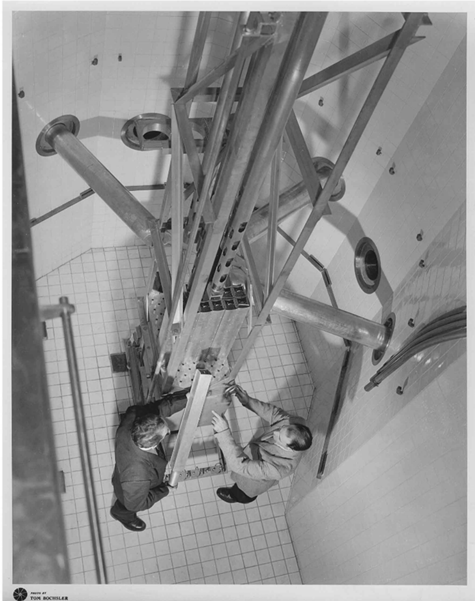
Figure 1-3: Overhead Photograph of the MNR Core. The man on the left is holding a fuel assembly (Photo courtesy of Tom Boschler).
