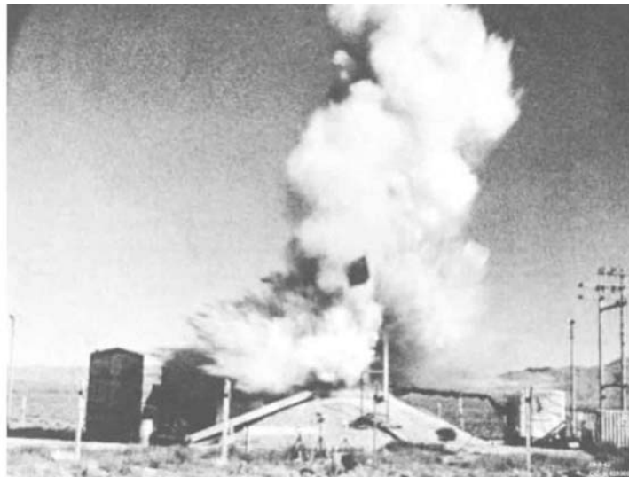
Figure 1-8: Steam and Water Expulsion from Borax I during the July 22, 1954 Destructive Test (Ref. 1-6)
