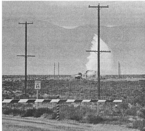
Figure 1-9: Steam and Water Expulsion from the Spert I Destructive Test on November 5, 1962 (Ref. 1-4)
